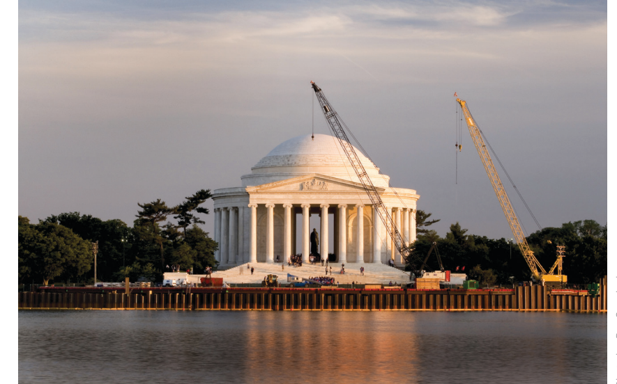
2008 Jefferson Memorial Seawall Repair
